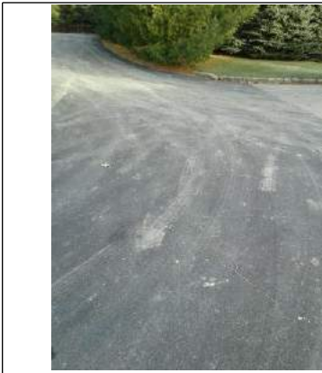
The blacktop driveway is in satisfactory condition.
