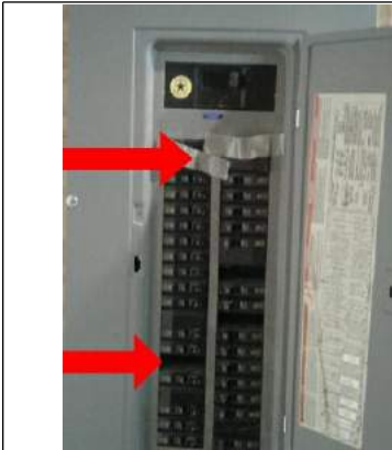
There are several missing Breakers in the Box. The Open Spaces should be filled in with blanks. The taped off Breakers at the top of the box we're for hot tubs which are no longer in the building.
